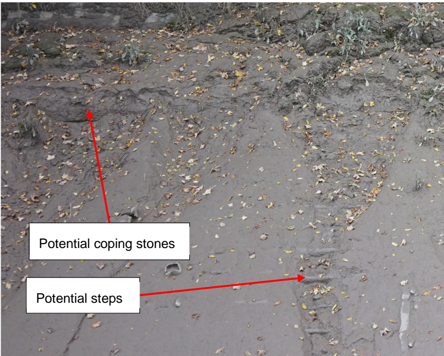
Figure 6.10: NCS06 Buried structure 2022
