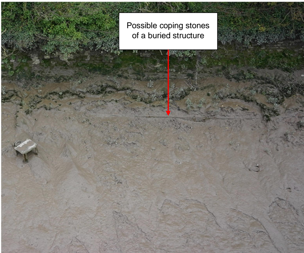
Figure 6.2: NCS06 Buried structure
